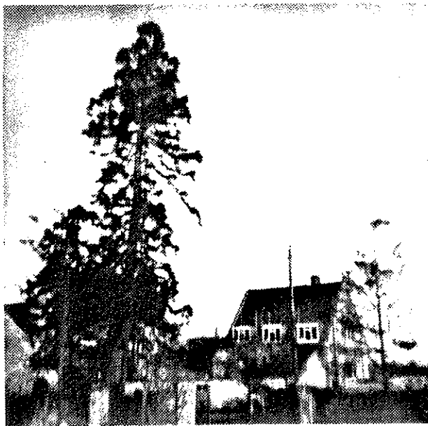
The Old Chapel being rebuilt as a dwelling- house in 1969.
